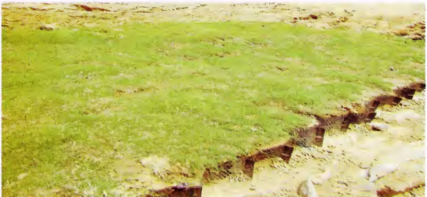
Fig. 15 Growth of Turfing on Embankment Side Slope after Application of Geocells
