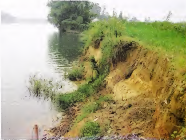
Fig . 7 Erosion of River Bank
