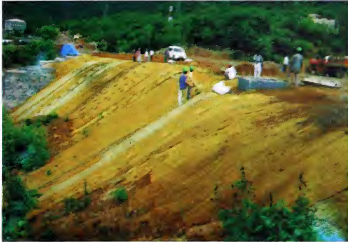
Fig. 12 Application of 3-D Mats on Denuded Road Side Slope
