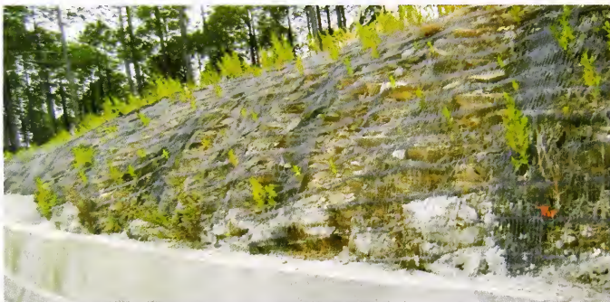
Fig . 11 Use of Synthetic Geogrids to Promote Vegetation on Barren Hill Slope
