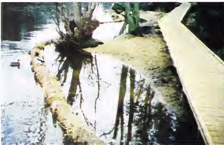
Fig. 18 Coir Fascines – Before and After Application of Coir Fascines
