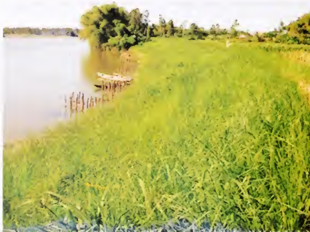
Fig. 8 Protection of the River Bank by Vetiver Grass
