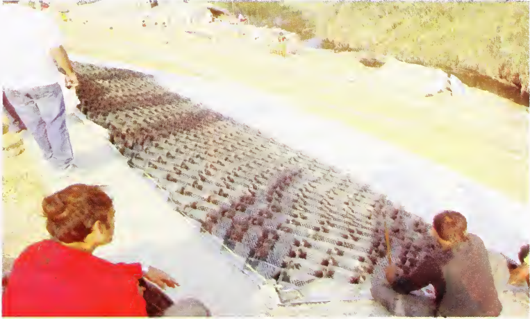
Fig. 14 Application of Geocells on Embankment Side Slope
