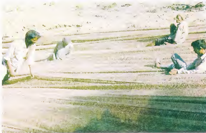
Fig. 9 Application of Jute Netting on Denuded Hill Slope
