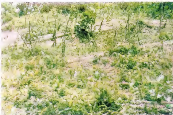
Fig. 10 Vegetation Growth after Application of Jute Netting and Sowing
