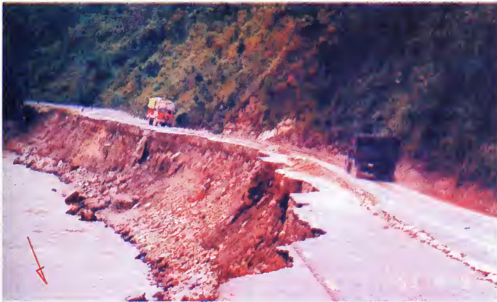
Fig. 6 Erosion of Road Embankment Adjacent to River
