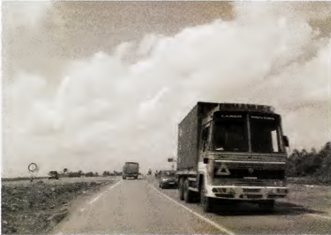
Fig. 29 : Condition of Completed Carriageway
