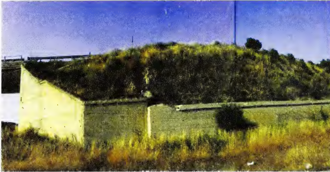
Fig. 20 : Completed Structure- S.Marco-Argentano Road Italy
