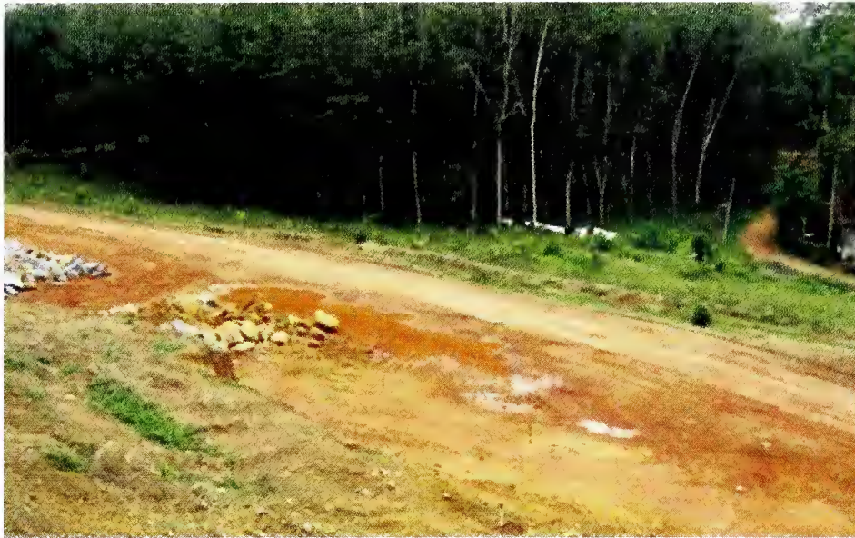
Fig. 15 : Seethawaka Industrial Park, Sri Lanka Site Before Construction
