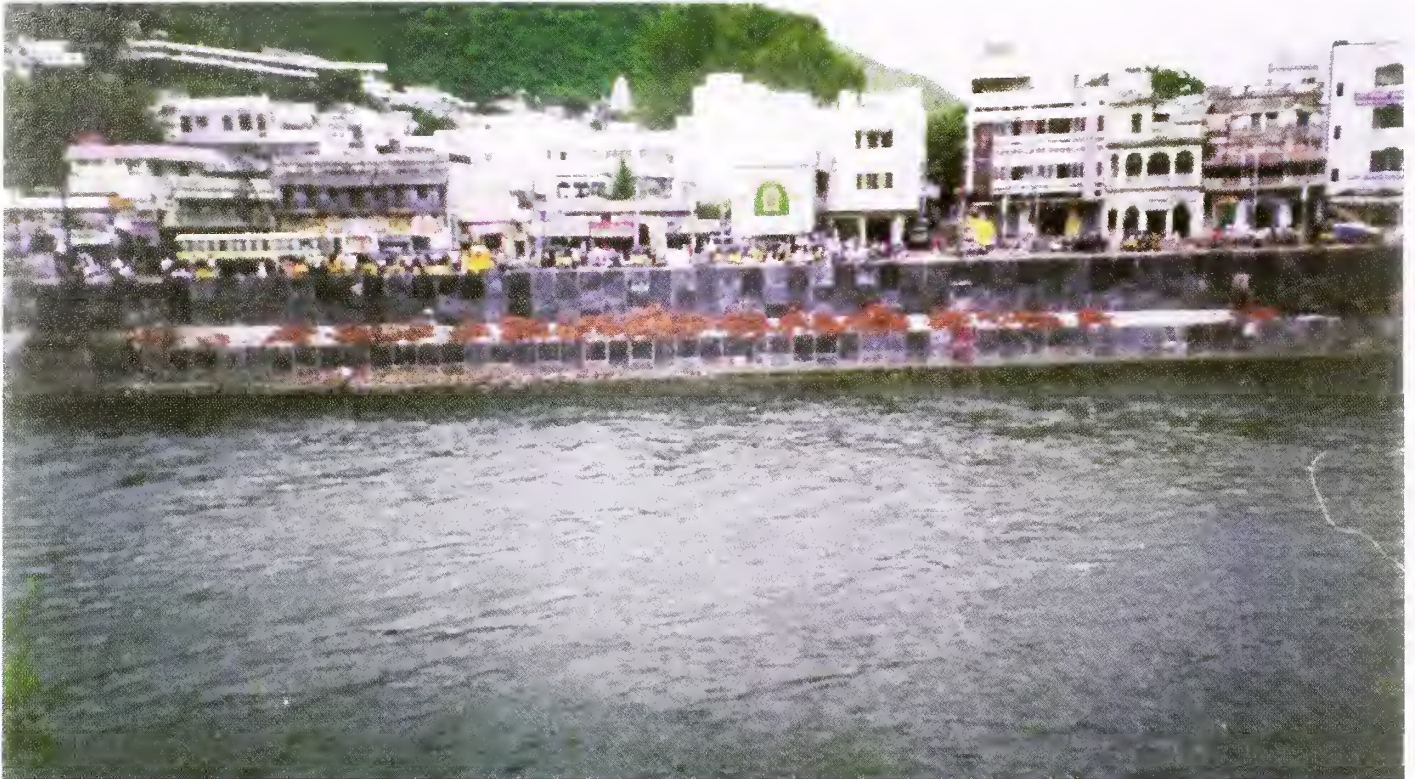
Fig. 35 : The Road Section After Completion of Restoration Works
