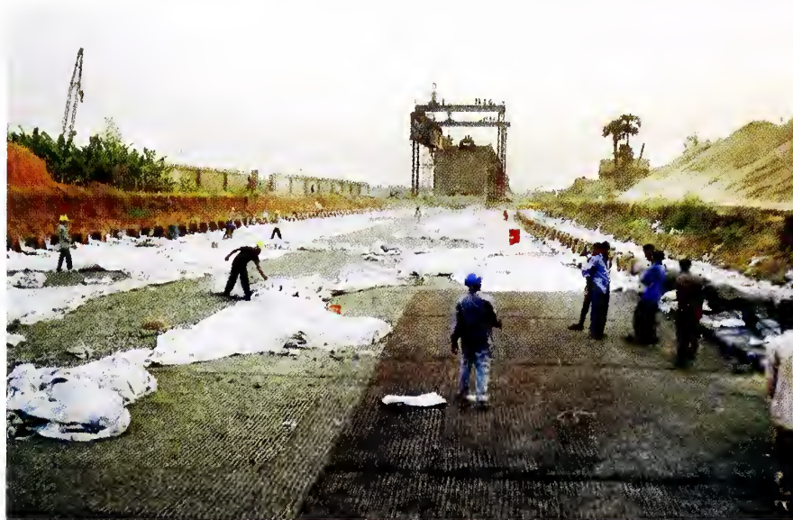
Fig. 23 : Construction of Basal Mattress at NH-5
