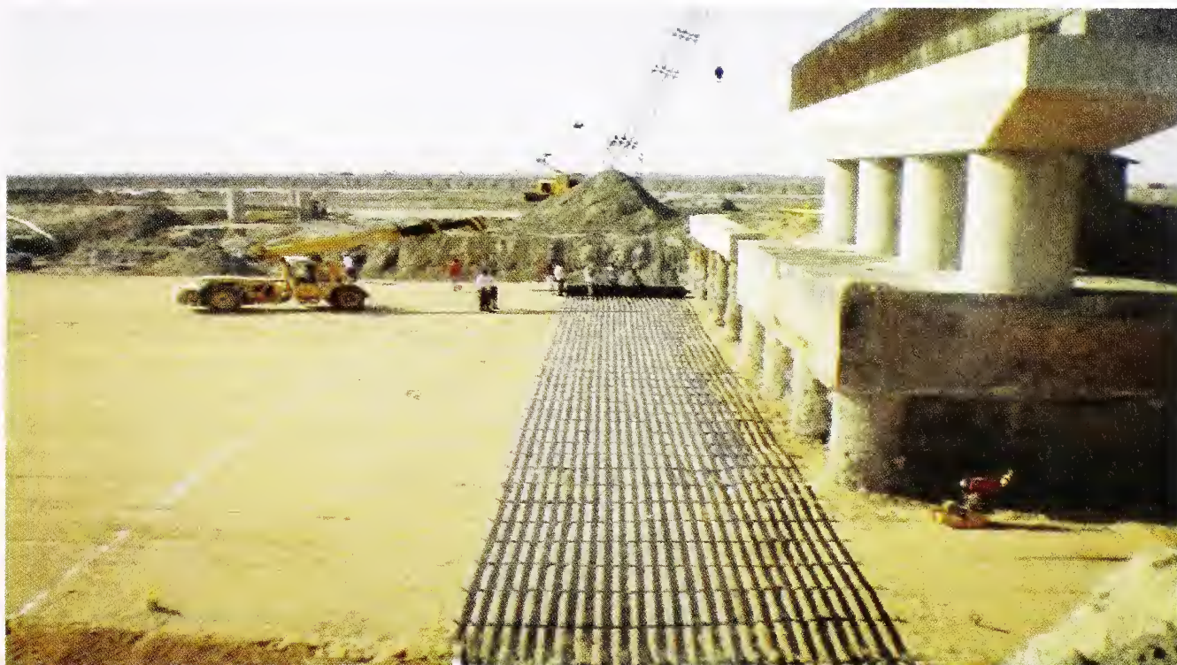
Fig. 28 : Installation of Bonded Geogrid, Mundra, Gujarat
