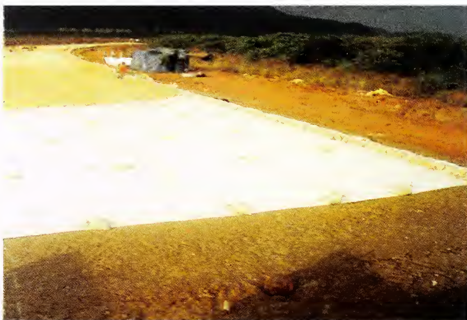
Fig. 25 : Geotextile as Basal Reinforcement at Visakhapatnam
