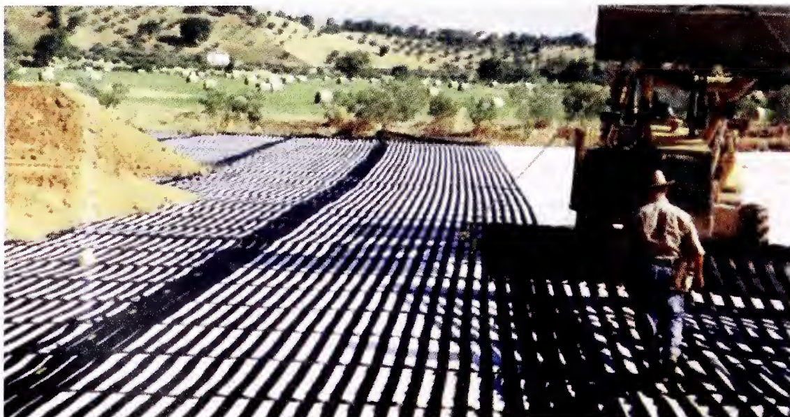
Fig. 19 : Installation of Bonded Geogrids Over Geotextile Separation Layer
