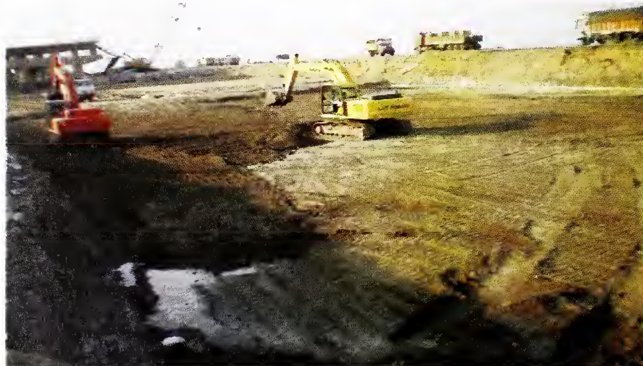
Fig. 27 : Installation of Drainage Layer, Mundra, Gujarat
