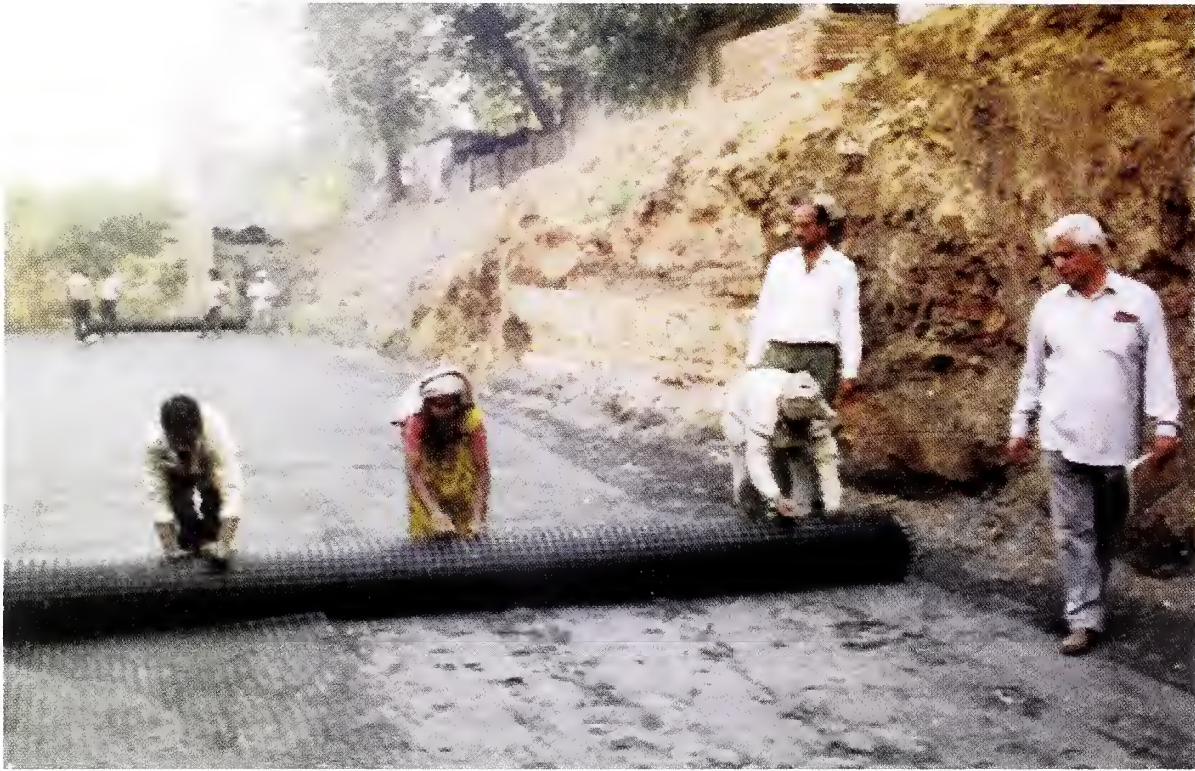
Fig. 32 : Spreading Geogrid as Basal Reinforcement at Okhla
