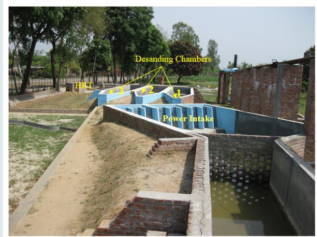
An Overview of the De-sanding Chamber Physical Model
