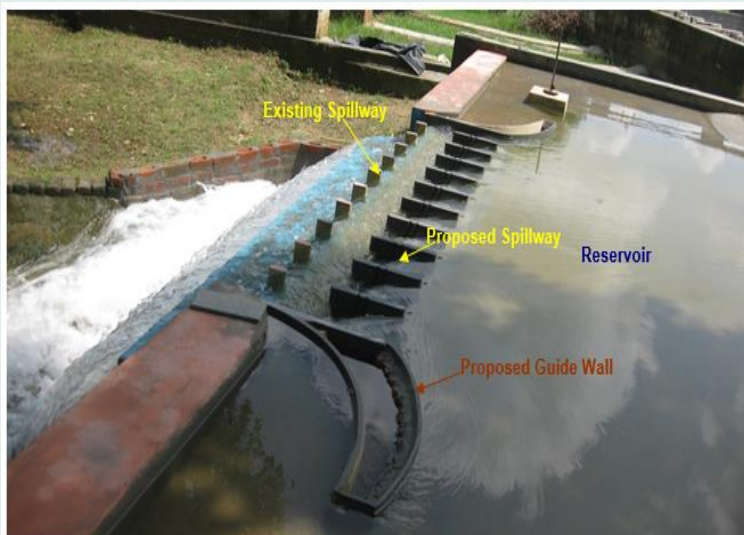
Side View of flow condition at 1,10,000 Cusec over Twin Spillways (Crest of Proposed Spillway at El 152.44 m)
