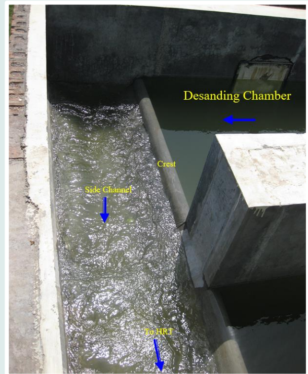
View of Flow Condition in the Side Channel
