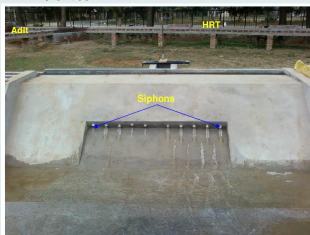
Siphonic Spillway in Operation
