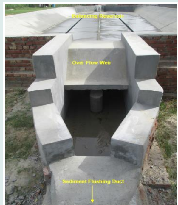
General View of Over Flow Weir
