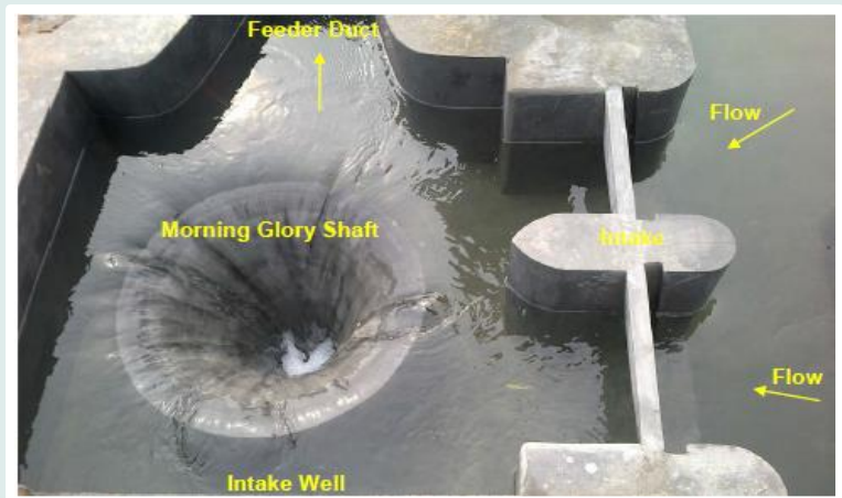
General View of the Intake Well with Morning Glory Shaft
