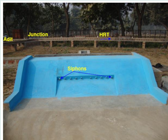
Front View of Siphonic Spillway
