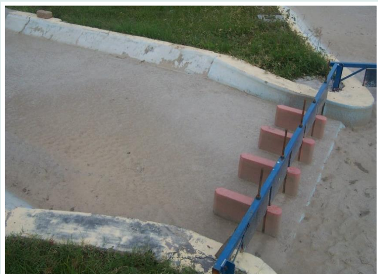
Sediment Deposition Pattern in Haidergarh Branch Final Proposal
