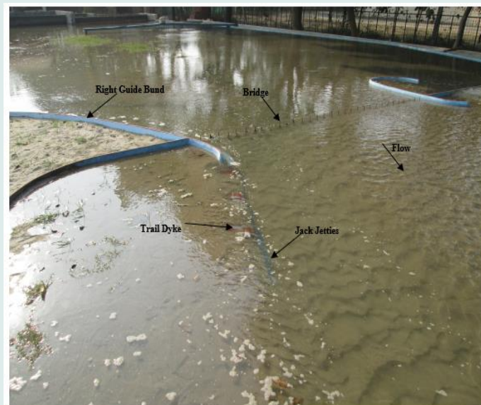
Flow Conditions with Trail Dykes and Jack Jetties D/S of Bridge at high flood discharge
