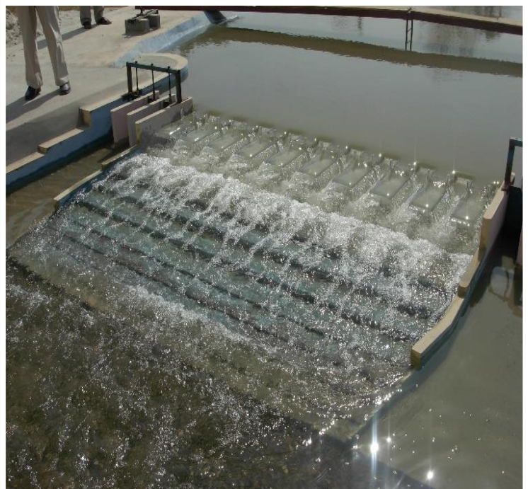
Running view of P. K. Weir from D/S with under sluice gate closed at 2500 m 3 /s discharge
