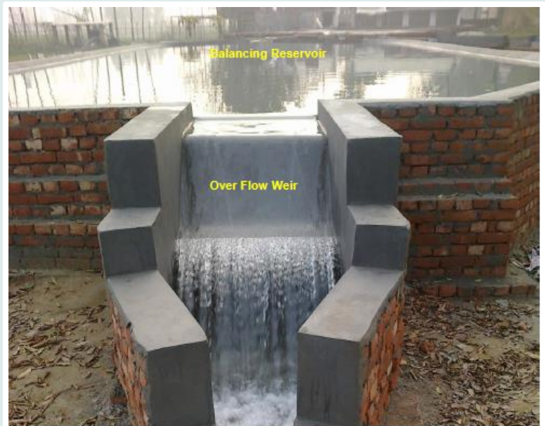
Flow at Over Flow Weir
