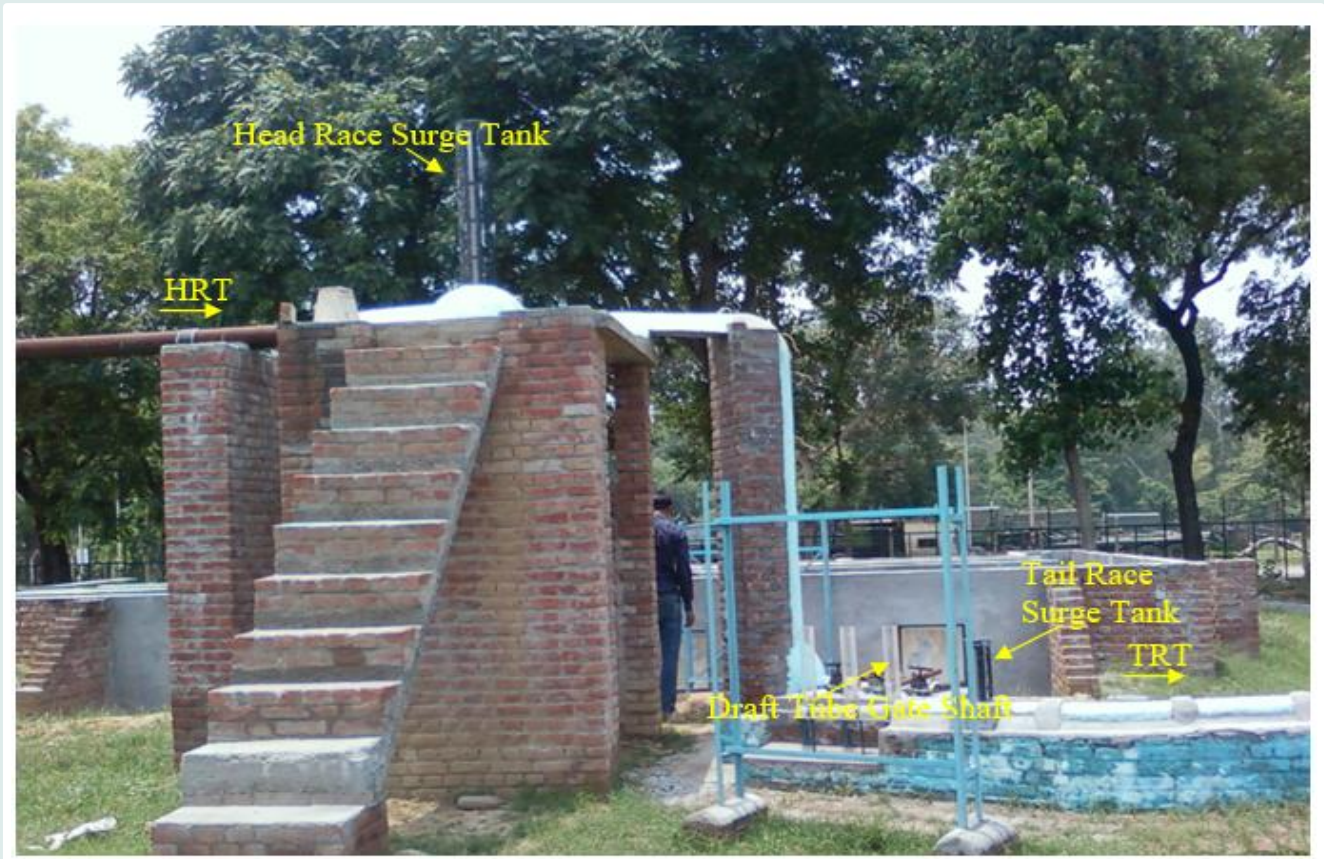
General View of the Surge Shaft and Tail Race Model
