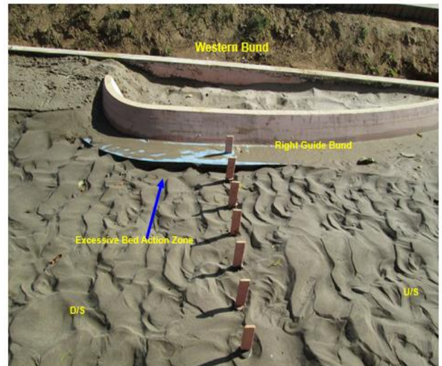
General View of Excessive Bed Action near Right Abutment
